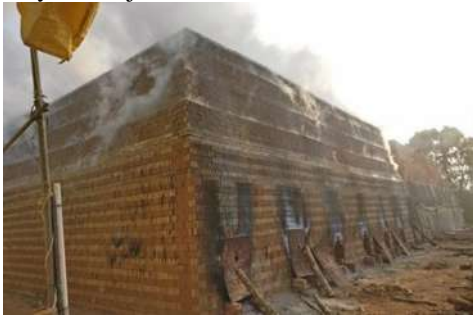
Fig-3: Bricks arranged for firing
