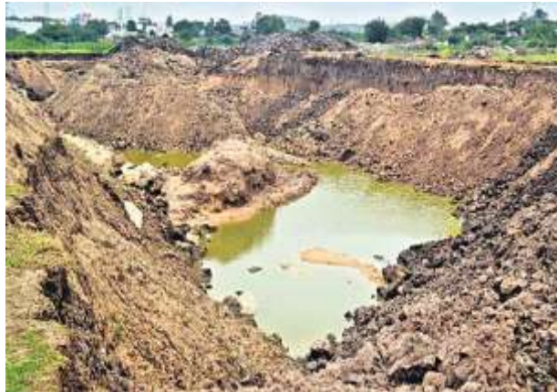
Fig. 2 Nala Dipping and Widening
