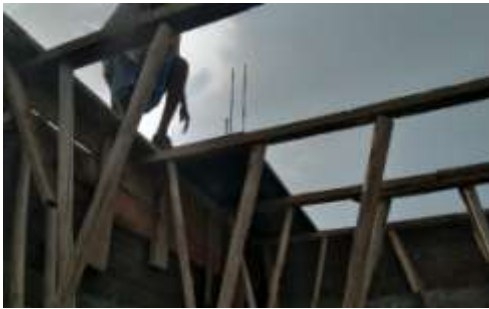
Building Roof-centring.
