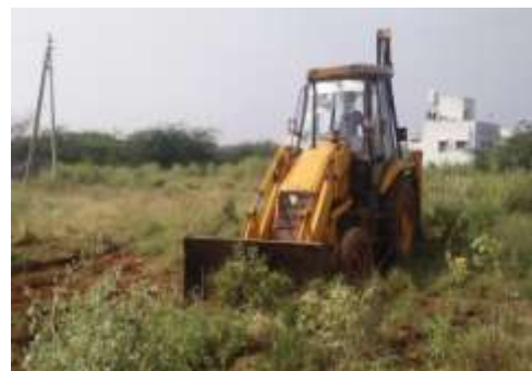
Site Leveling and Prepration
