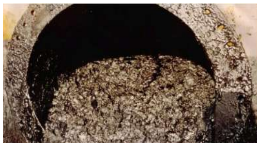
Fig 4. oil tank bottom sludge
