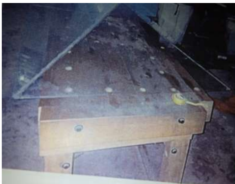
Figure:1. Tetrahedral Glass top Under Construction
