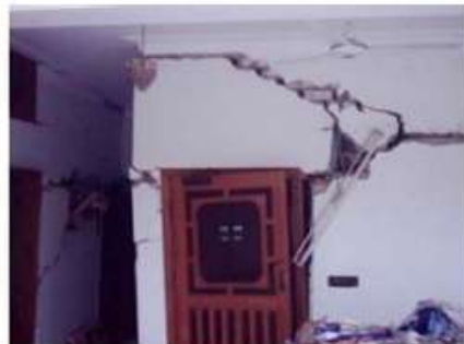
Fig. 1: Combined in-plane and out-of-plane failure mode in Kashmir 2005 (Naseer et al. 2010)
