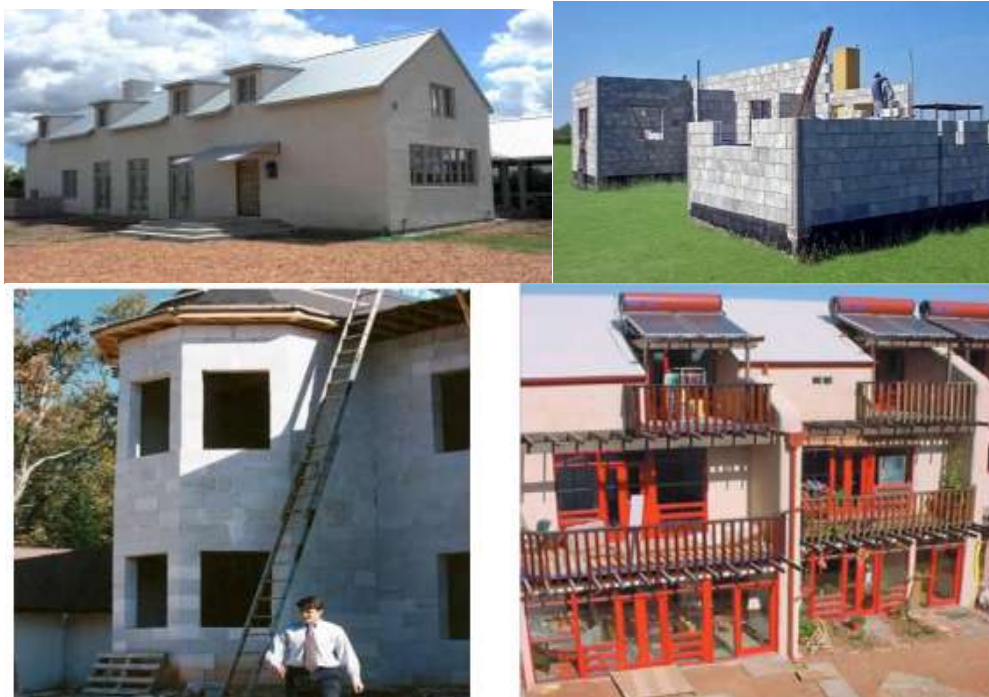
Fig 5: Unreinforced AAC structures
