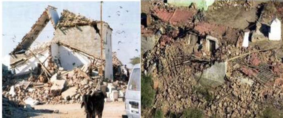
Fig.7: Bhuj earthquake damage to URM, 2001
