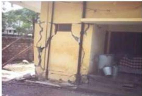
Fig. 1: Combined in-plane and out-of-plane failure mode in Kashmir 2005 (Naseer et al. 2010)
