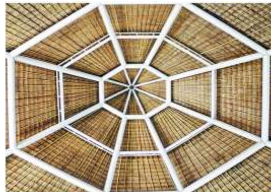
Figure-3 Bamboo Roof
