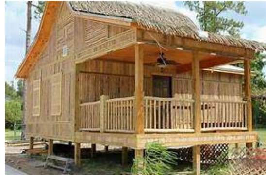
Figure-1 Bamboo House
