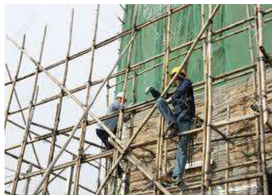
Figure-4 Bamboo Scaffolding
