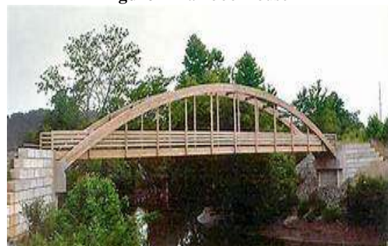
Figure-2 Bamboo Bridge
