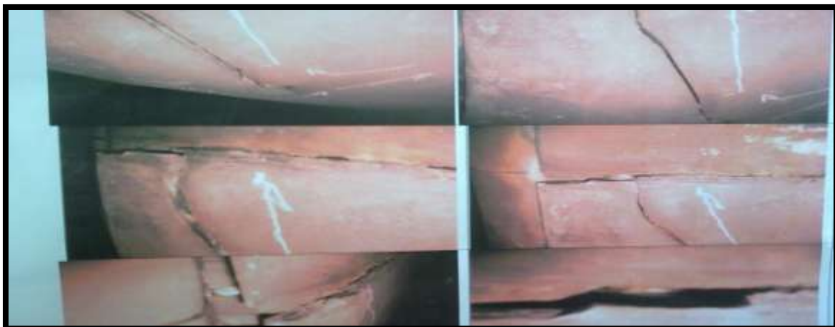
Fig (4) show the crack of (HGC).
