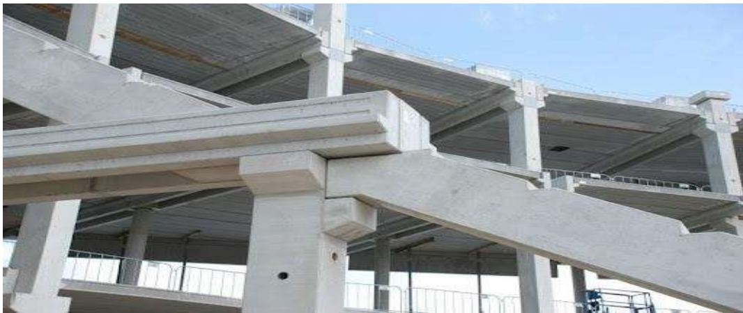
Fig: ARTIFICIAL READYMADE BEAMS AND COLUMNS
