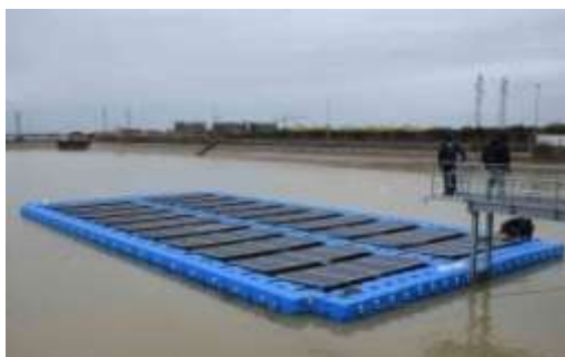
Surface Mounted Floatovoltaics
