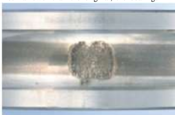
a. Pitting on the inner rings in ball bearings
