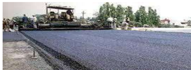
Figure.3. Roads made with plastic waste
