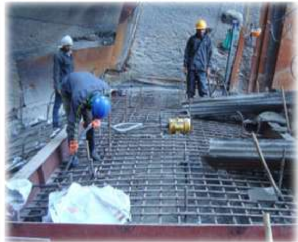
Photograph 6: (Laying concrete in spillway bay no 2)
