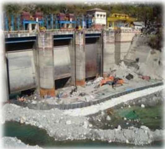
Photograph 5: (Temporary Bund for channelization of stream water)
