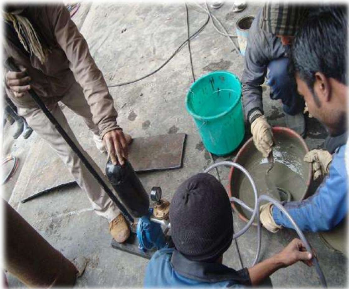
Photograph 7: Laying and Grouting of MS Plate in Spillway Bay no 2
