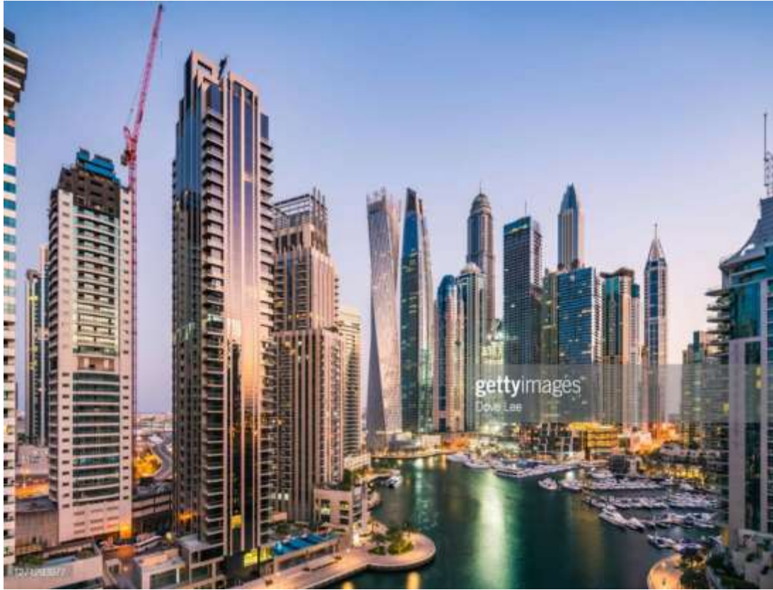
Figure 6: View of Marina One from the top
