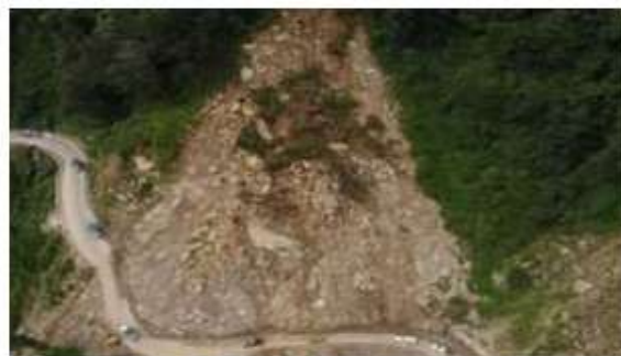
Figure 1: Typical slide zone along road
