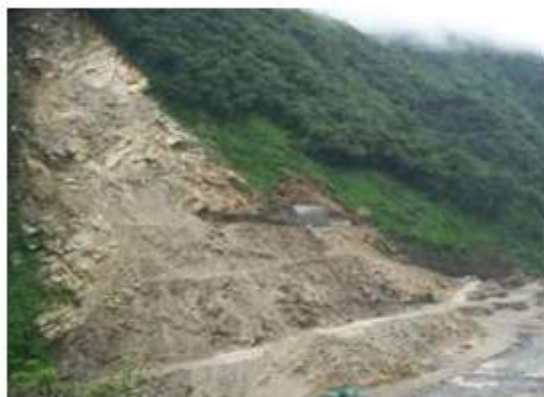
Figure 5: Site condition before start of work
