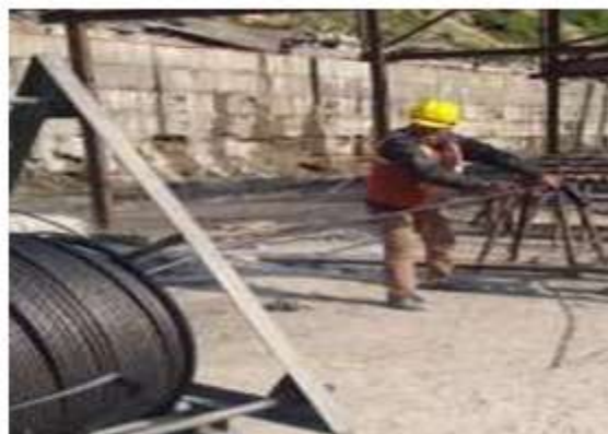
Figure 6: Before commencement of cable anchoring
