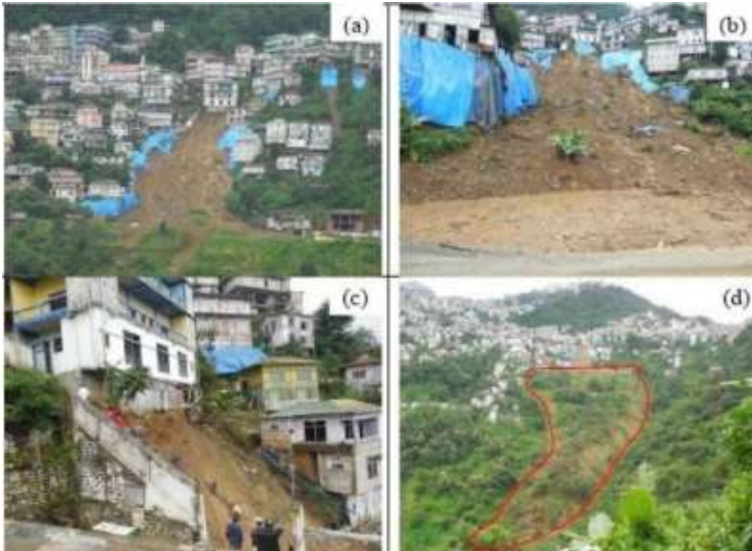
Fig. 1: (a) Distant view of Hunthar Venj landslide (b) Closure view of Hunthar Venj landslide (c) Main scarp of slide (d) Distant view of landslide with toe erosion due to two flowing streams at the bottom meeting a common stream.
