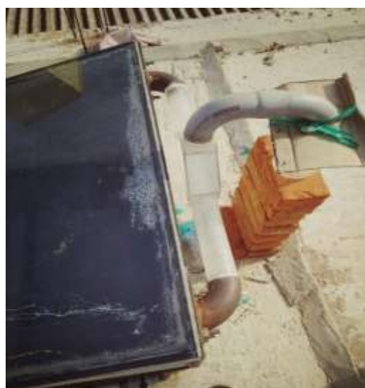
Fig. 6 Process Operation after the installation of Chimney
