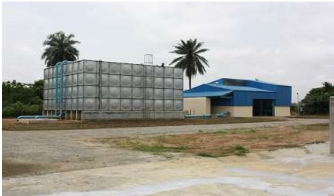
2 Plate. 5: Temporary Water Supply System
