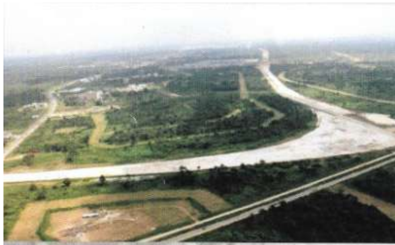
Plate.6: Construction of Internal Township Roads
