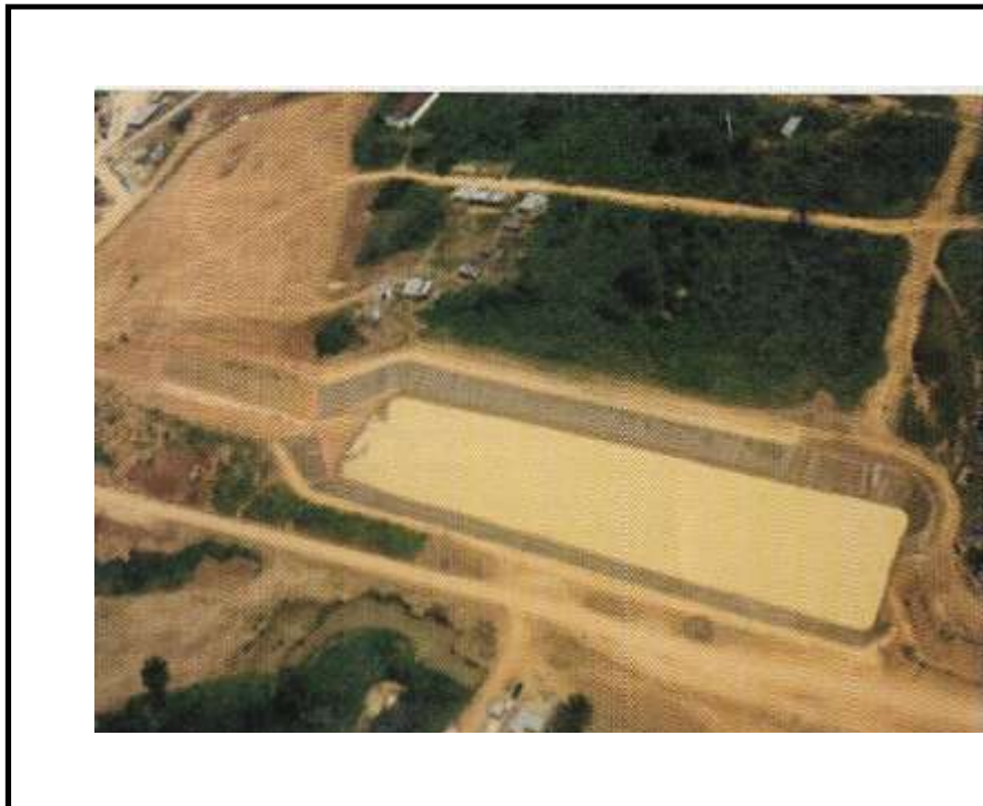
Plate. 3: Emergency Bulk Storm Water Canal Detention Pond
