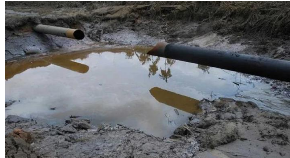
Figure 6: Pipeline vandalism Source: NNPC, 2019
