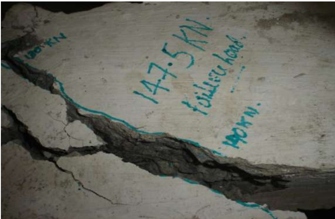
Fig. 11 Close view of the crack in Beam 1 after failure
