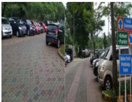
Fig [6] and [7] Conblocks used for pavement of Parking area [25]
