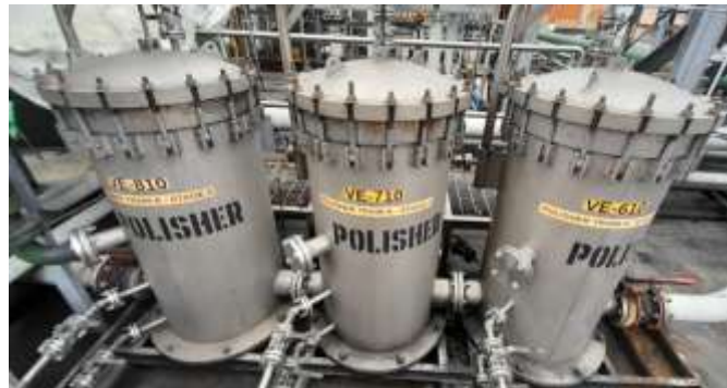
Figure 5: Jones Creek Produced water treatment Polishers train(courtesy: researcher JC field visit)
