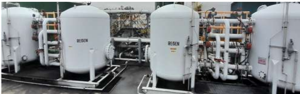
Figure 4: Regen water treatment unit (courtesy: researcher JC field visit)
