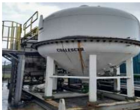
Figure 3: Pictorial view of a produced water treatment Coalescer unit (Courtesy: researcher JC field visit)
